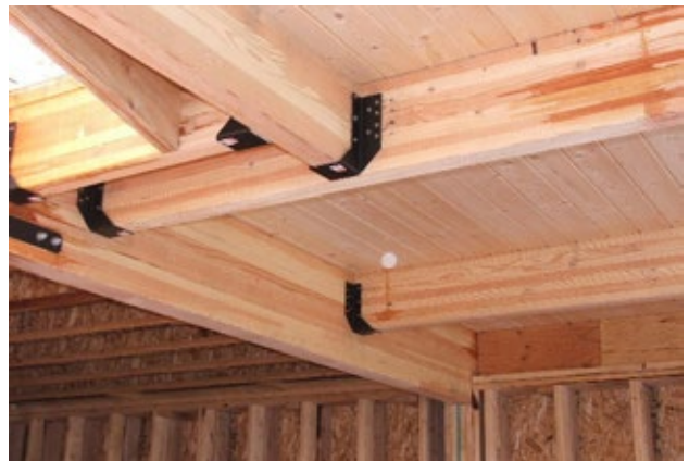
FIGURE 5.2: MASS TIMBER CONNECTOR EXAMPLES
