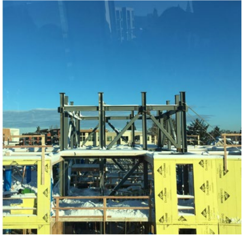
FIGURE 6.18: TIMBER FRAME AND STEEL CORE PROGRESSING IN COLD, SNOWY WEATHER
