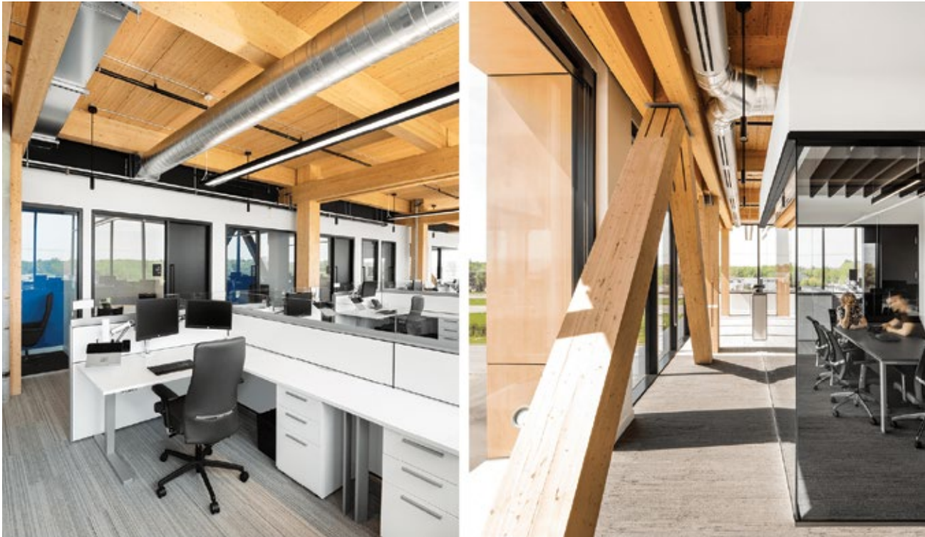
FIGURE 6.3: POST AND BEAM BUILDING
