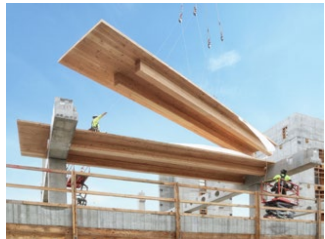
ABOVE AND RIGHT — FIGURE 6.9: COMPOSITE TIMBER AND PRECAST CONCRETE STRUCTURE
