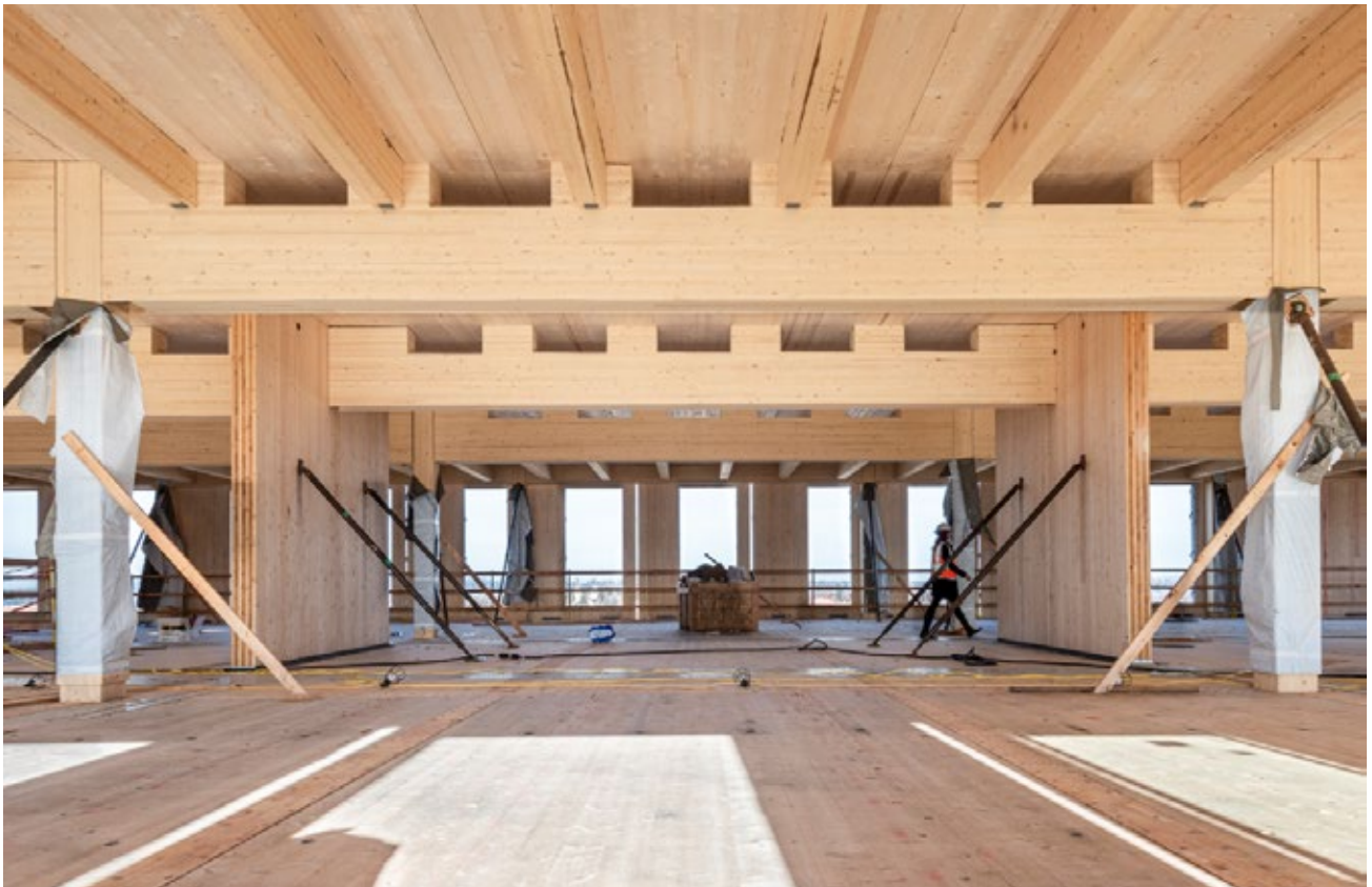
TOP LEFT – FIGURE 5.13: POST TENSIONED TIMBER BEAM
