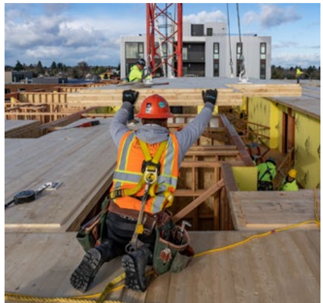
FIGURE 6.8: A SMALL FRAMING CREW GUIDES PANEL PLACEMENT
