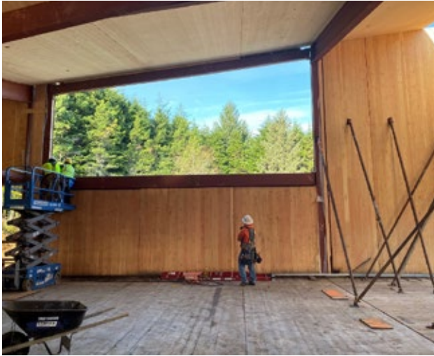
FIGURE 6.10: CLT WALL AND ROOF PANELS WITH STEEL FRAMING
