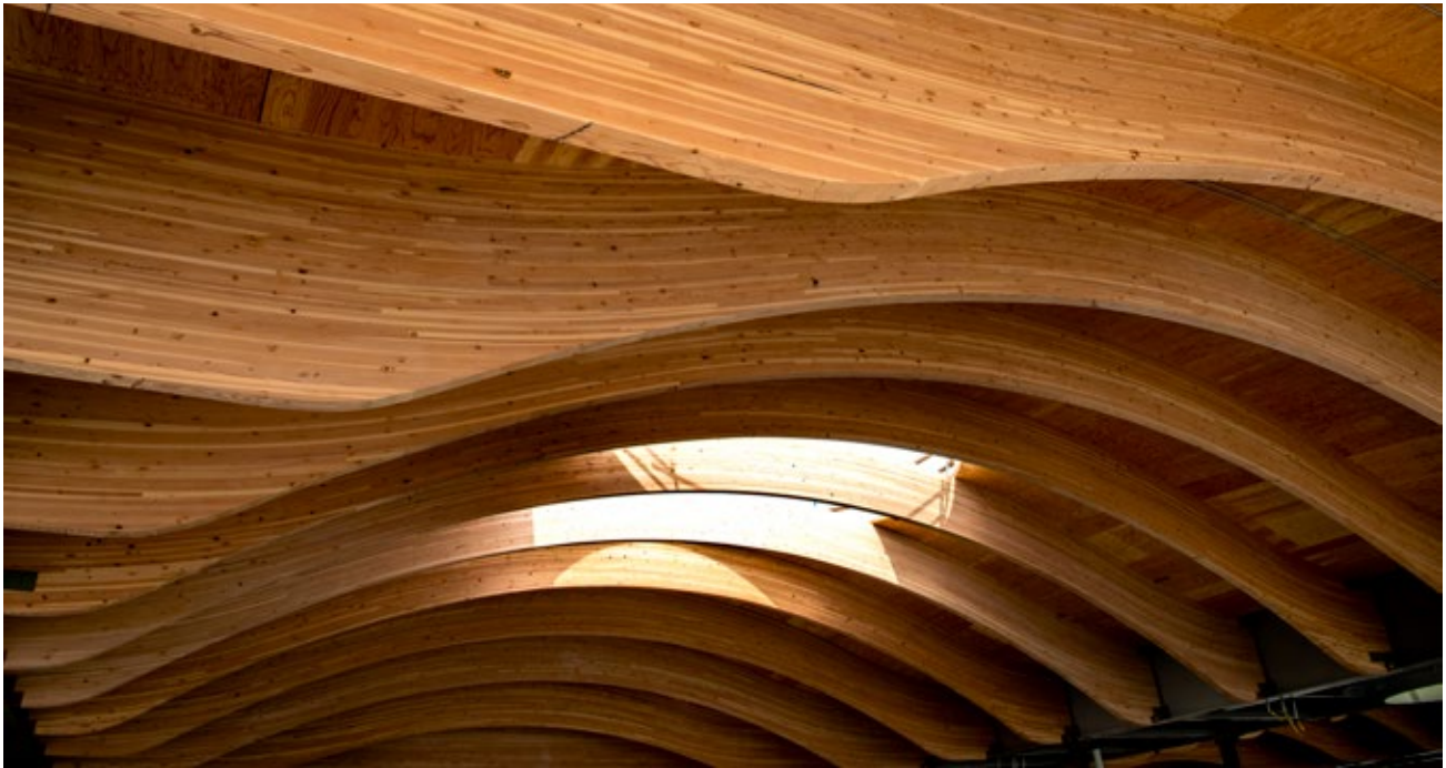
WOODEN ROOF OVER PDX'S NEW MAIN TERMINAL
