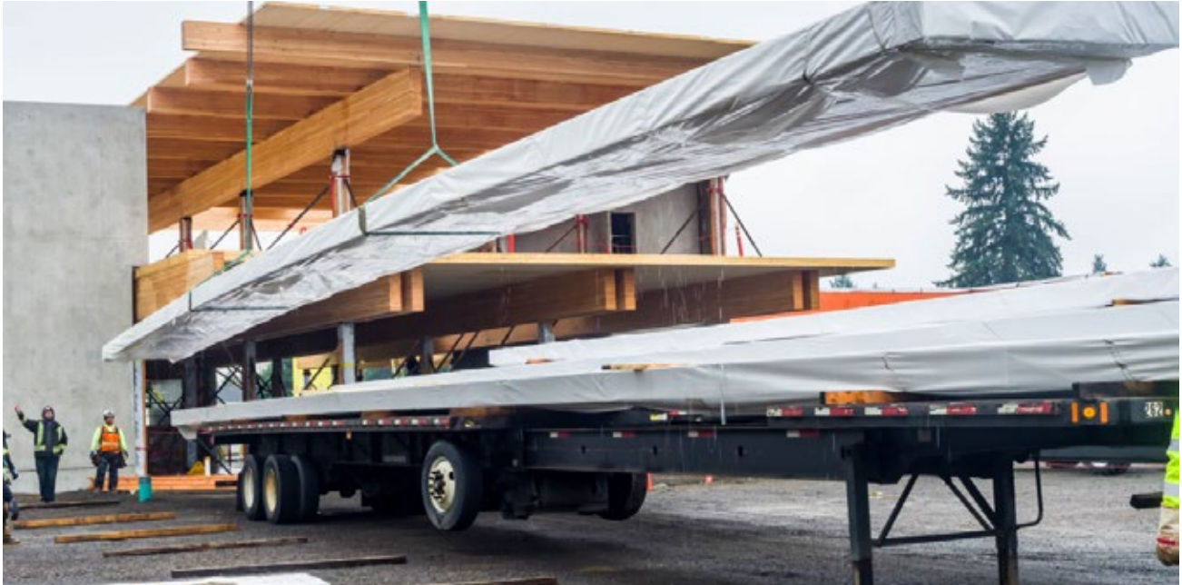
FIGURE 6.20: CLT PANELS PROTECTED WITH WRAP FOR TRANSPORT AND ON-SITE STORAGE
