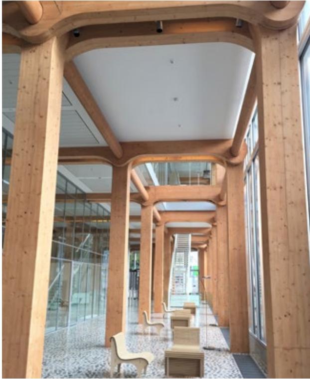
FIGURE 5.3: CNC JOINERY WITH PREFABRICATED MASS TIMBER COLUMNS AND BEAMS
