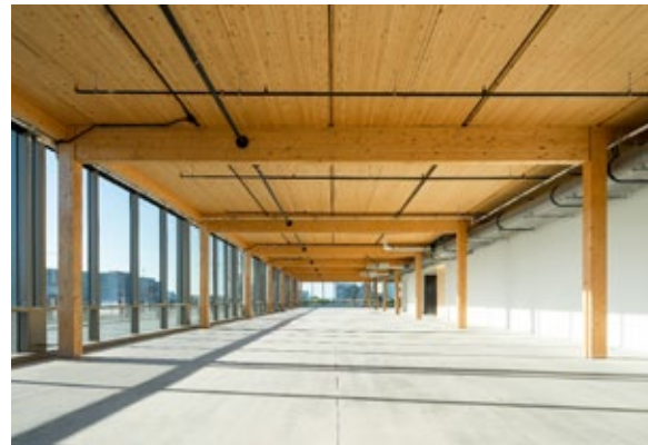
FIGURE 3: INHERENTLY, 2-BY-8 DLT HAS A 38 SOUND TRANSMISSION CLASS (STC) RATING. BUT WITH THE ADDITION OF A ¾-INCH ACOUSTI-MAT AND 3-INCH TOPPING SLAB, THE STC CAN EXCEED 50. THAT HELPS MITIGATE NOISE FROM ABOVE AND FORMS A CREATIVE SPACE FOR SINGERS AND SONGWRITERS.
