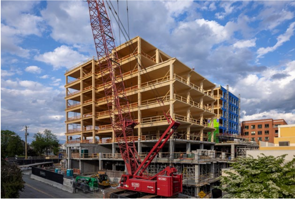
APEX PLAZA DURING CONSTRUCTION Photo Credit: Prakash Patel Photography
