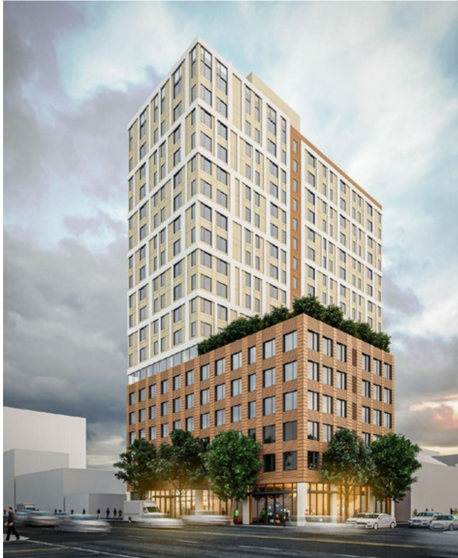
RENDERING OF OWOW'S 19-STORY AFFORDABLE HOUSING PROJECT. FRERES ENGINEERED WOOD'S MASS PLY PANELS WERE SELECTED FOR THEIR EFFICIENT, SUSTAINABLE, EASY-TO-INSTALL, AND COST-EFFECTIVE ATTRIBUTES.
