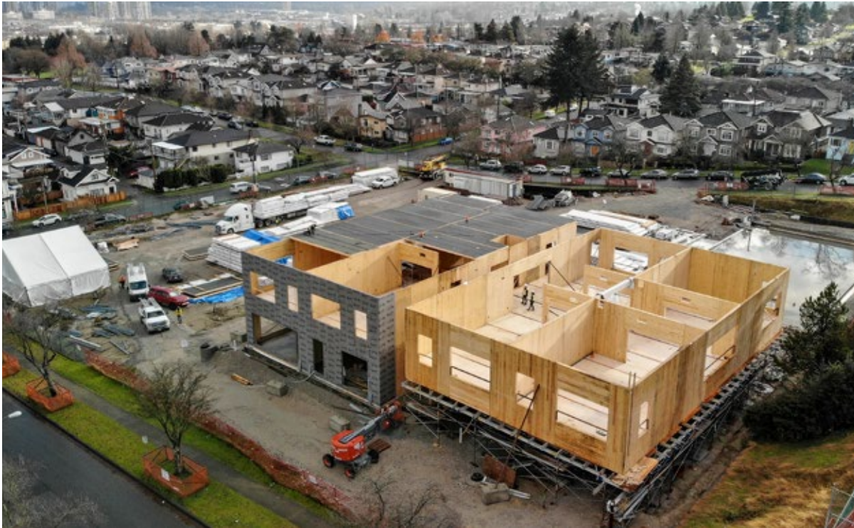
SIR MATTHEW BEGBIE ELEMENTARY SCHOOL UNDER CONSTRUCTION
