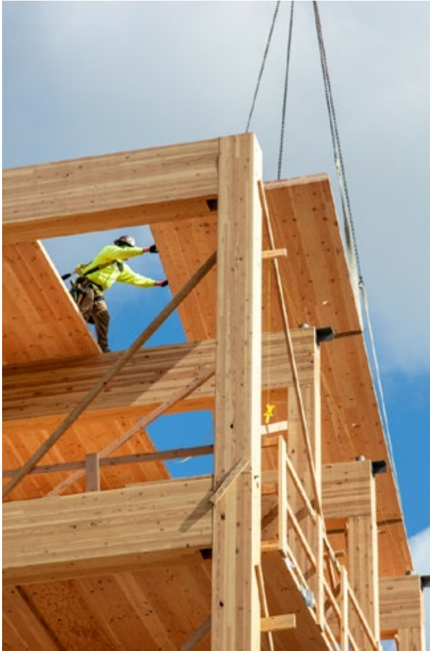
FIGURE 6.16: CRANE LIFTING WITH SLINGS
