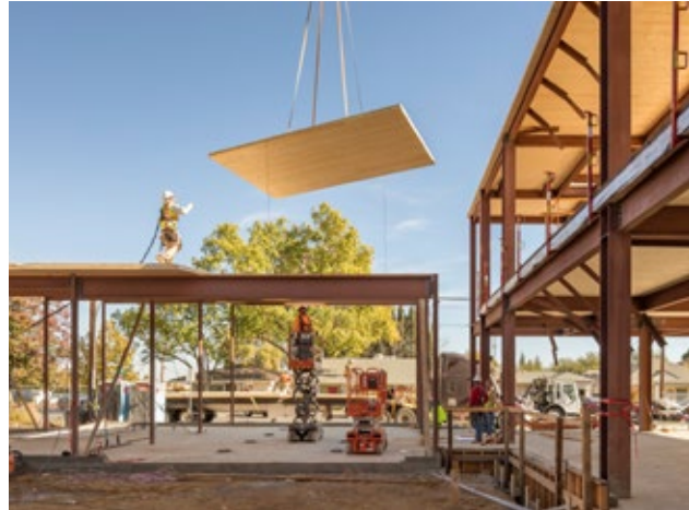
FIGURE 6.11: CLT FLOOR DECKS WITH STEEL FRAMING
