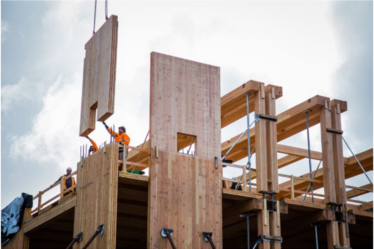
FIGURE 5.19: POST-TENSIONED CLT 'ROCKING' SHEAR WALL INSTALLATION
