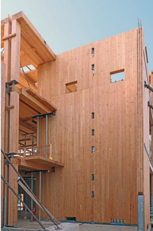
FIGURE 8.10: CLT ROCKING SHEAR WALL
