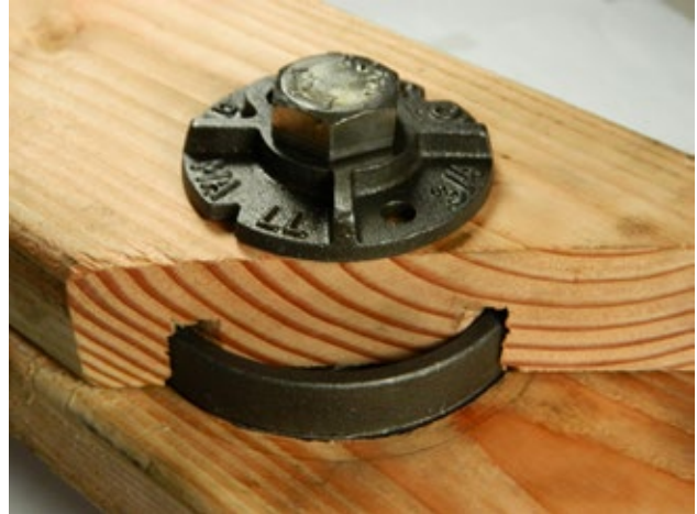
FIGURE 5.6: SHEAR PLATE CONNECTOR
