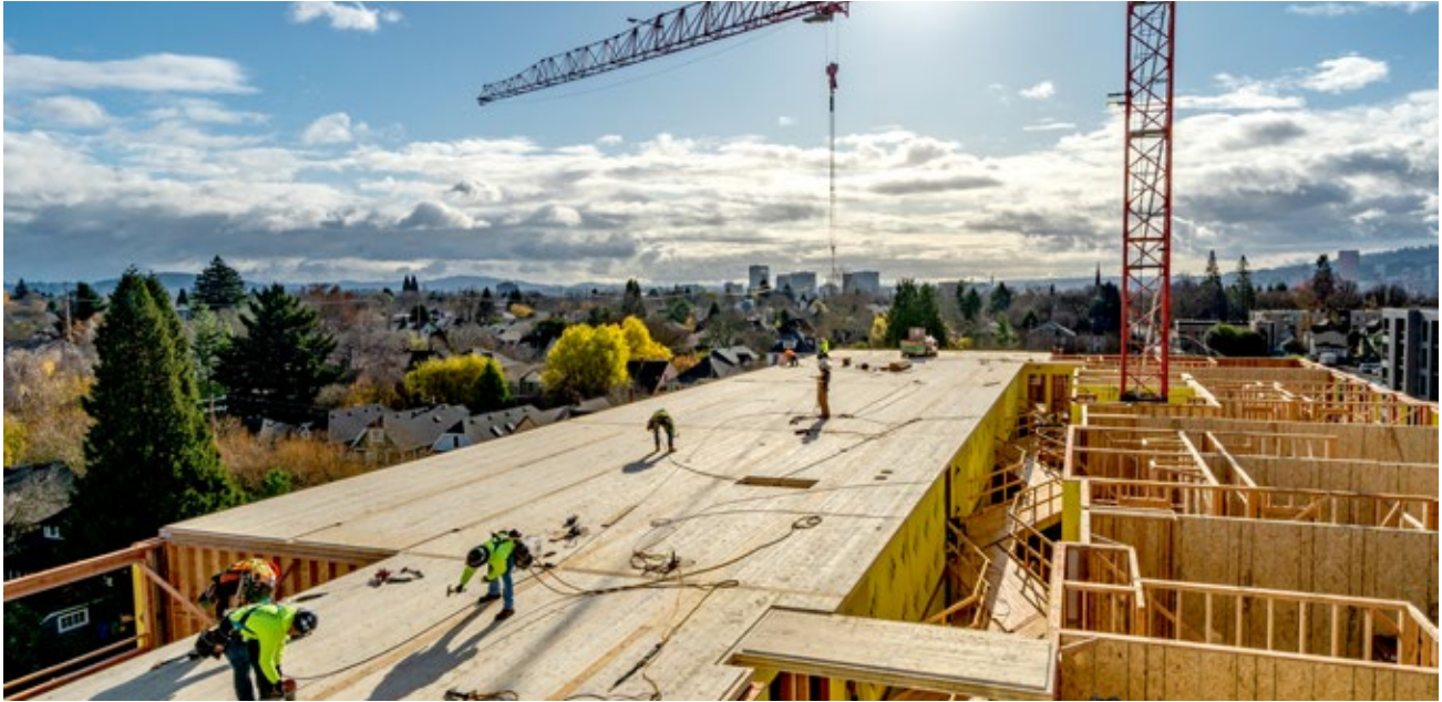
FIGURE 5.16: LIGHT FRAME AND MASS TIMBER HYBRID
